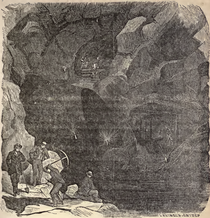
IN THE WEST JORDAN MINE.
