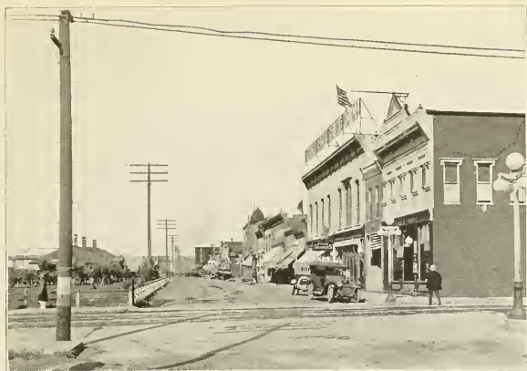
SOUTH FRONT STREET, ROCK SPRINGS
