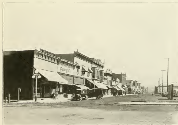
NORTH FRONT STREET, ROCK SPRINGS
