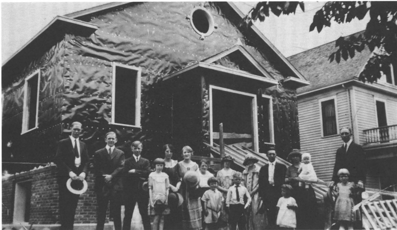
Members of the Minneapolis Branch in front of the Fourteenth Avenue chapel, under construction in 1924.
