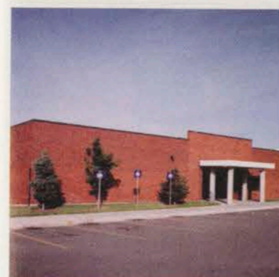
UTA TIMPANOGOS FACILITY OPERATIONS & MAINTENANCE
